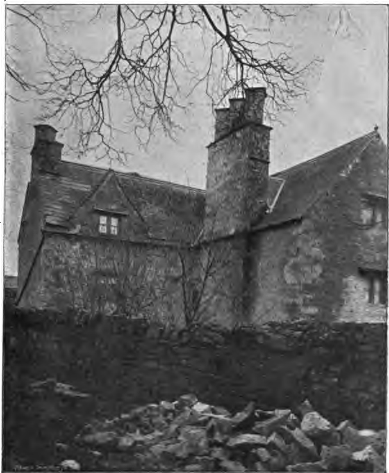
FIG. 2.—BACK OF HOUSE AT ABERTHUN, COWBRIDGE.
